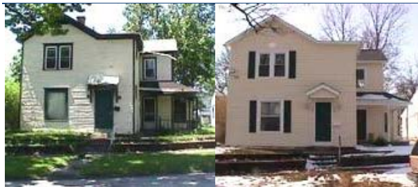
A CHIP Rehabilitation Project before (Left) and after (Right)
